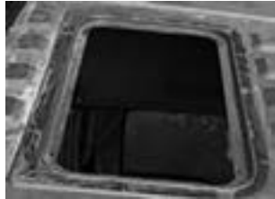
STEP 1 - Removing the skylight.
